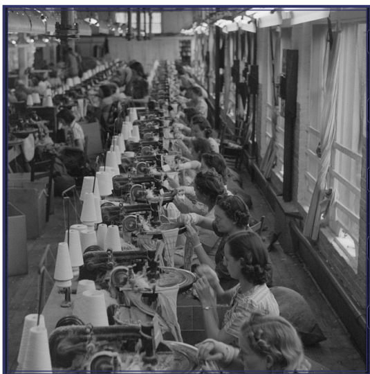
Figure 8. Inside of Union Point Hosiery Mill in 1941
