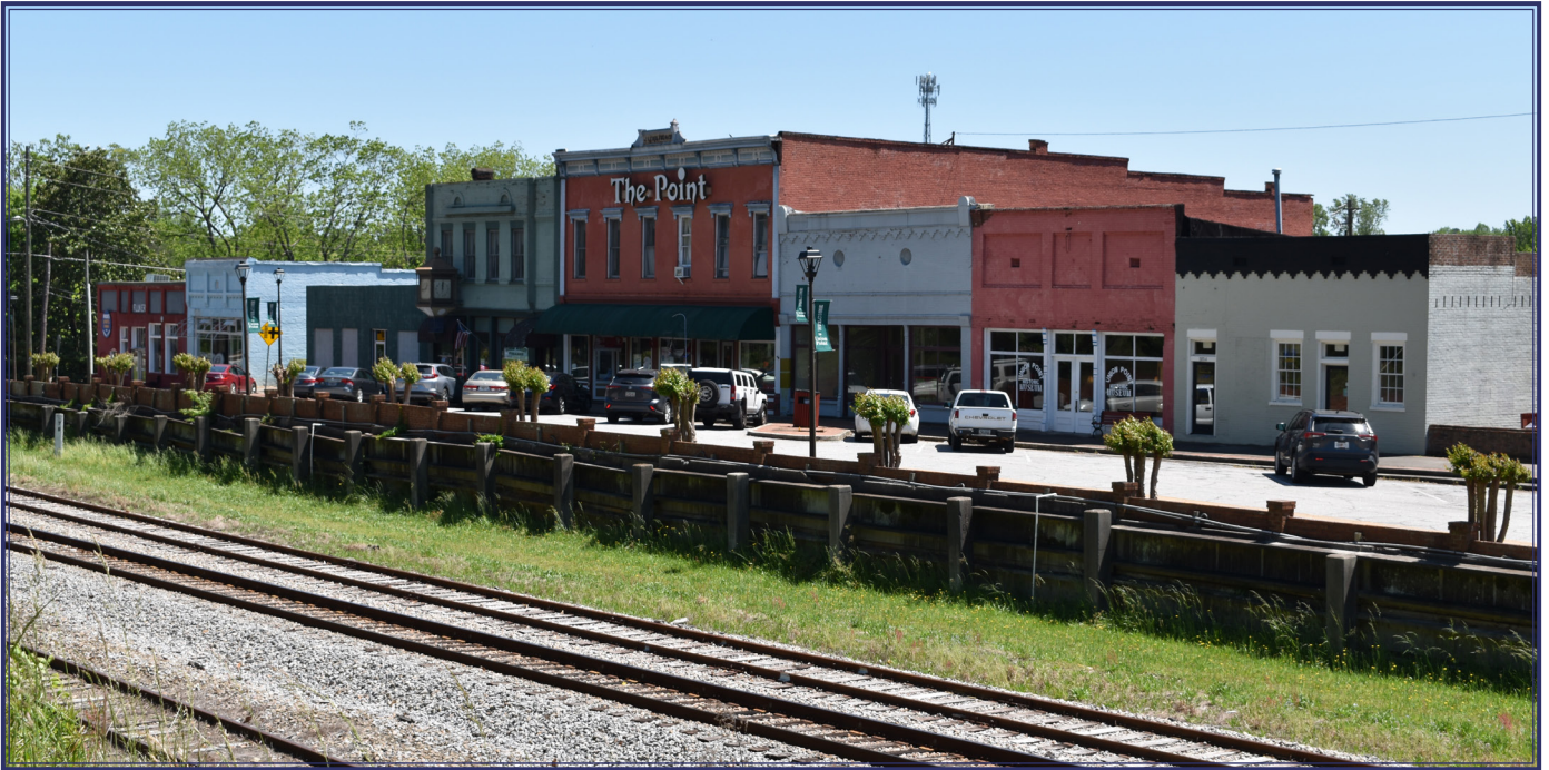
Figure 26. Downtown Union Point, as viewed from Wayside Park across the railroad tracks
