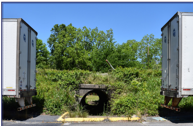
Figure 25. A passage under the railroad track connecting Union Manufacturing Company with the Historic Mill Village
